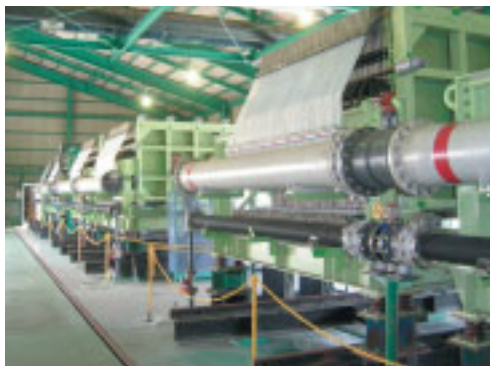
Yokkaichi Complex Electrolysis Plant
