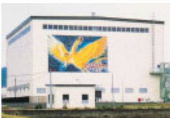
The RDF facility in Shunan City The Phoenix is a mythical bird that symbolizes rebirth and new life.
