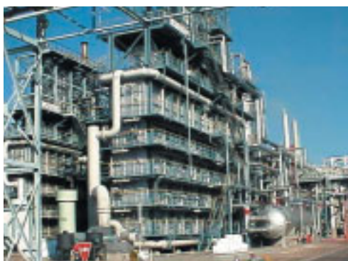
VCM plant at the Nanyo Complex
